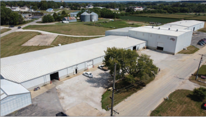
Jacobs manufacturing plant for pellet mill replacement parts as well as our die and roll shell rework department
