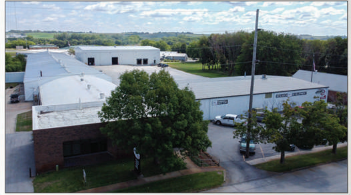
Jacobs general office and manufacturing plant for hammermill replacement parts
